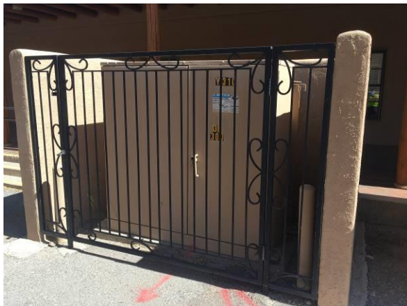
Photo #15 View of one of three pad-mounted transformers located in the southern and northern portions of the site.
