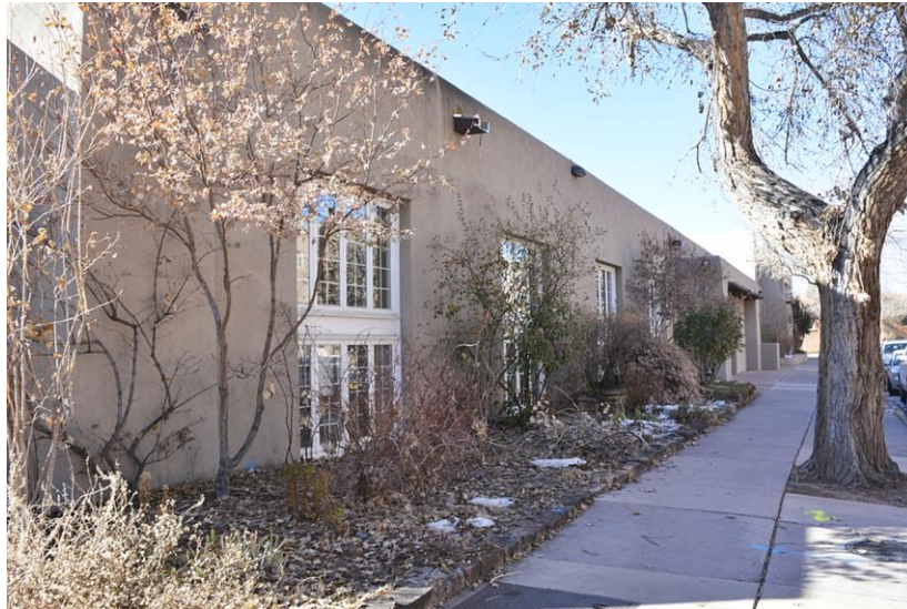
Photo 2: North elevation, 1942 building Camera facing southwest.
