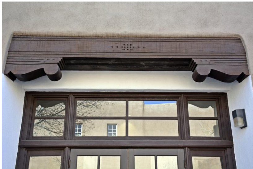
Photo 11: North elevation, 1950 addition, corbelled beam over entrance. Camera facing up.
