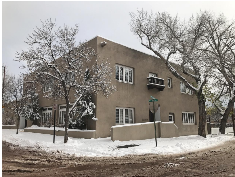
Photo 13: West elevation, 1950 addition. Camera facing southeast. November 28, 2019.
