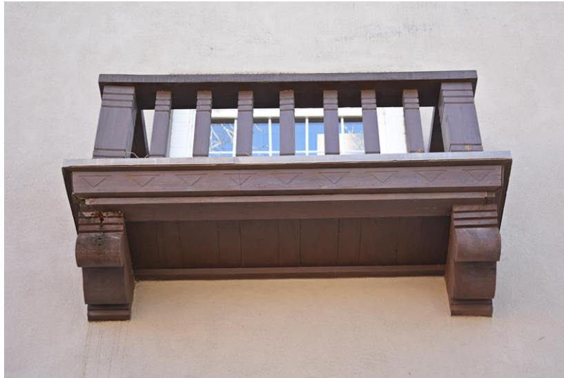
Photo 14: West elevation, 1950 addition, balconette. Camera facing up.
