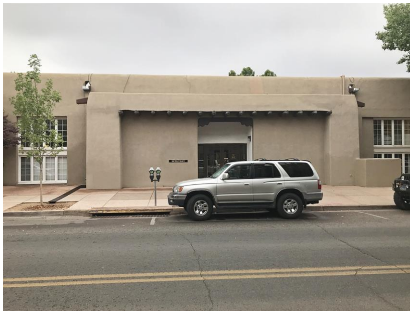
Photo 3: North elevation, 1942 building. Modified entry at center. Camera facing south. July 1, 2019.
