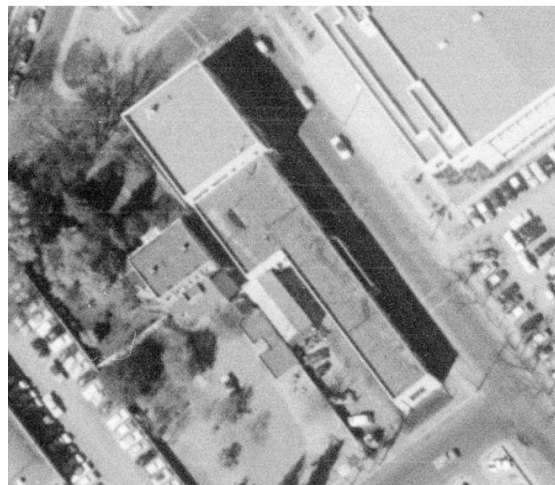
Figure 20: 1958 aerial photograph. Note gabled workshop at site of current parking lot. Courtesy NMDOT.
