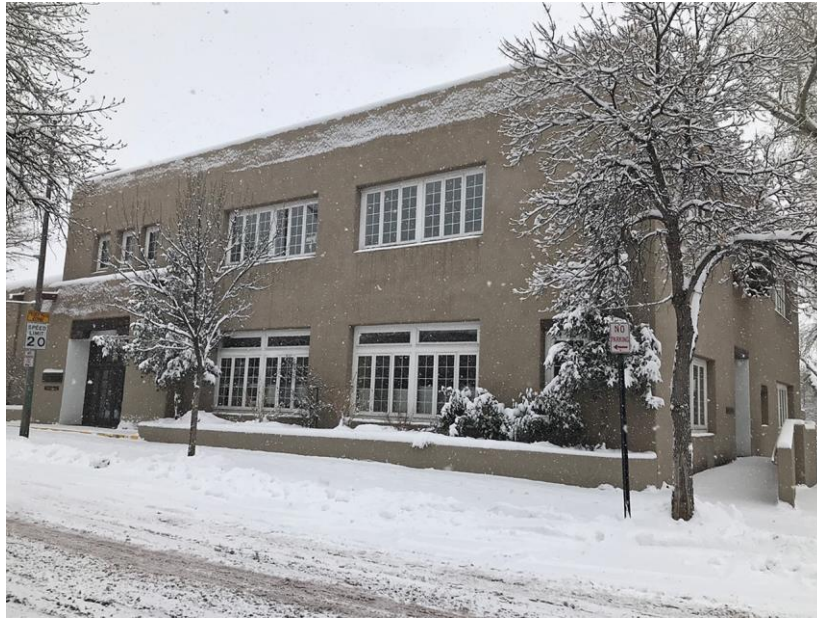
Photo 12: North elevation, 1950 addition. Camera facing southeast. November 28, 2019.
