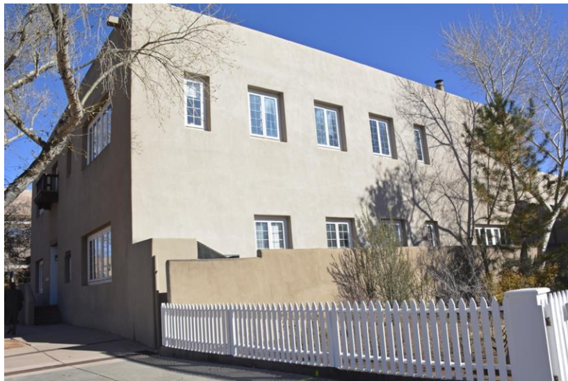
Photo 15: South elevation, 1950 addition. Camera facing northeast.
