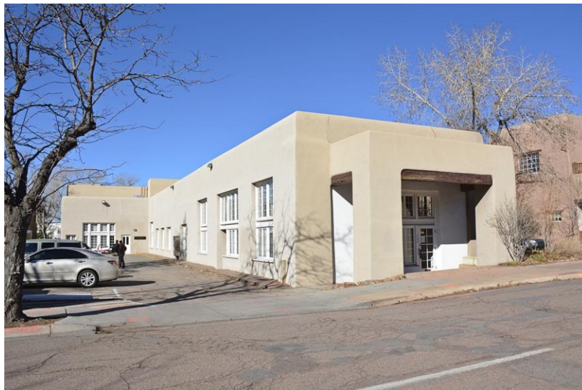
Photo 5: East and south elevations, 1942 building. Camera facing northwest.
