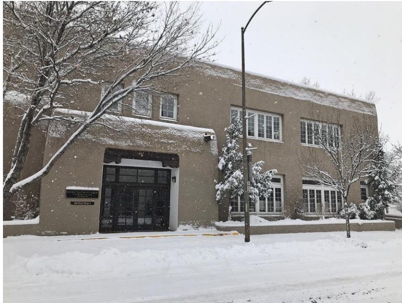
Photo 10: North elevation, 1950 addition. Camera facing southwest. November 28, 2019.
