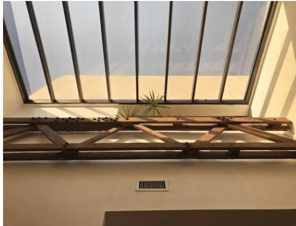
Photo 18: Skylight and surviving truss, 1942 building. Camera facing up.
