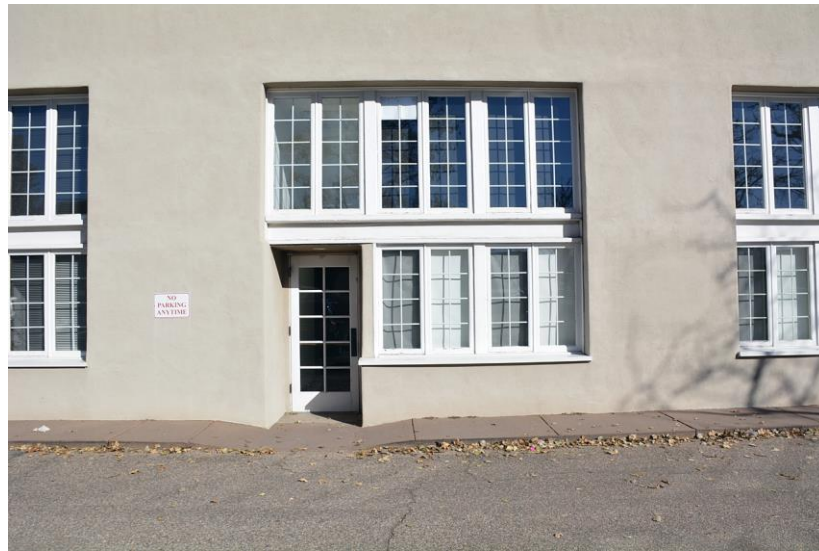
Photo 6: South elevation, 1942 building. Infilled overhead door opening. Camera facing north.
