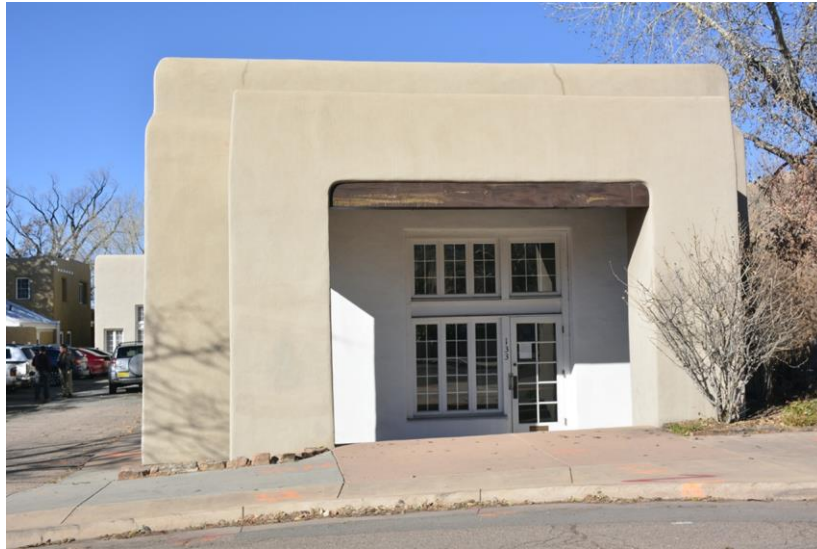
Photo 4: East elevation, 1942 building. 1979-80 portal at center. Camera facing west.
