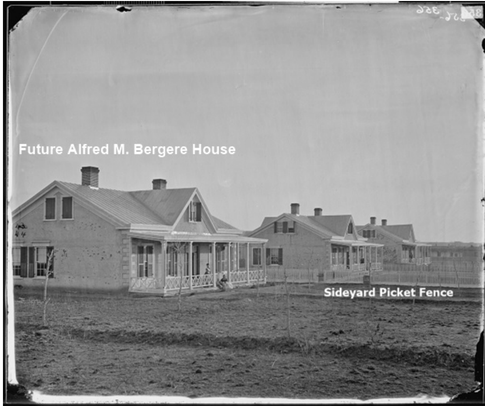
Figure 6: Future Alfred M. Bergere House, c.1873. North and west elevations.
