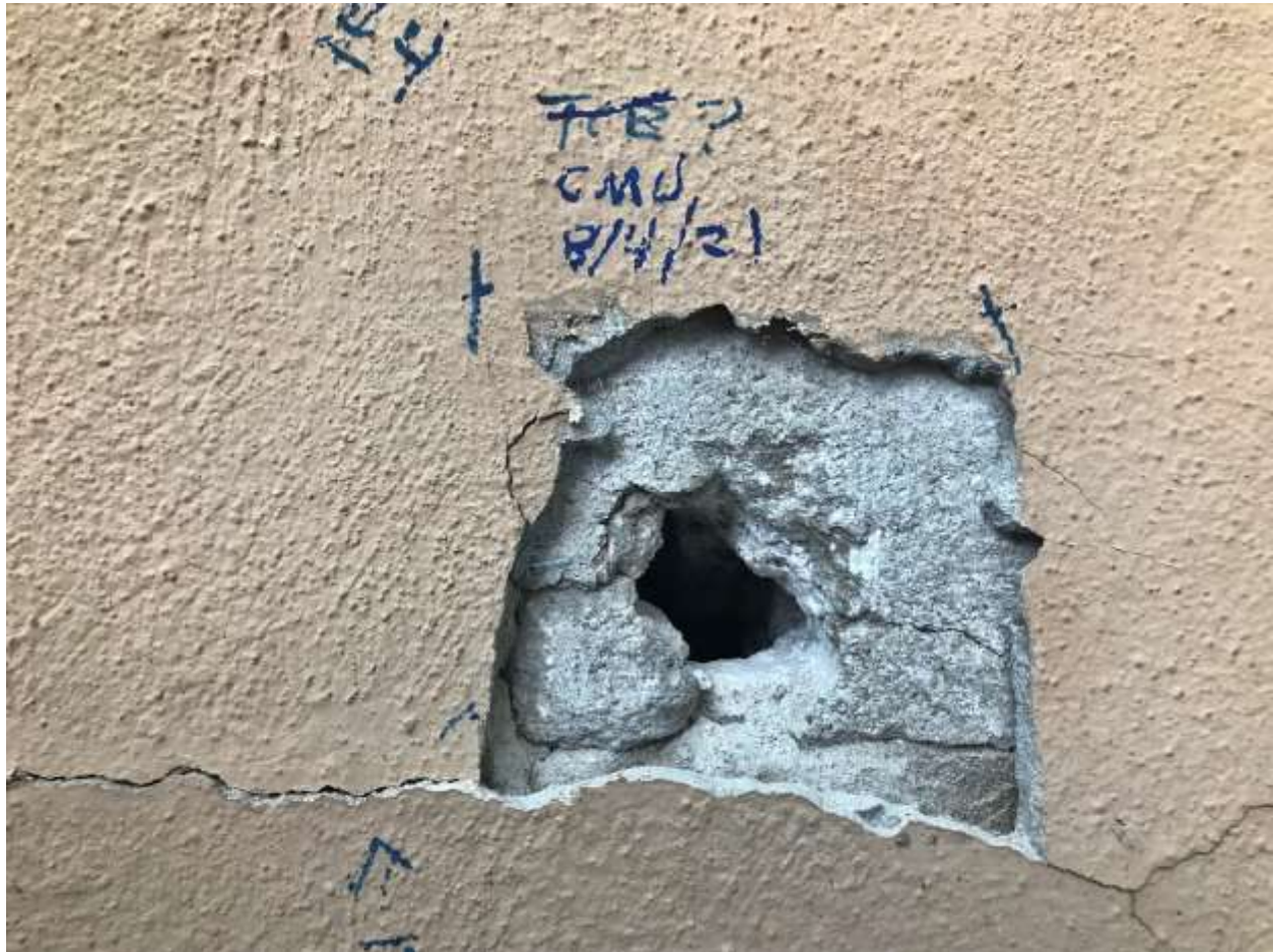
Figure 25: Test bore #4, “Middle Section,” showing CMU construction. August 4, 2021, John W. Murphey.
