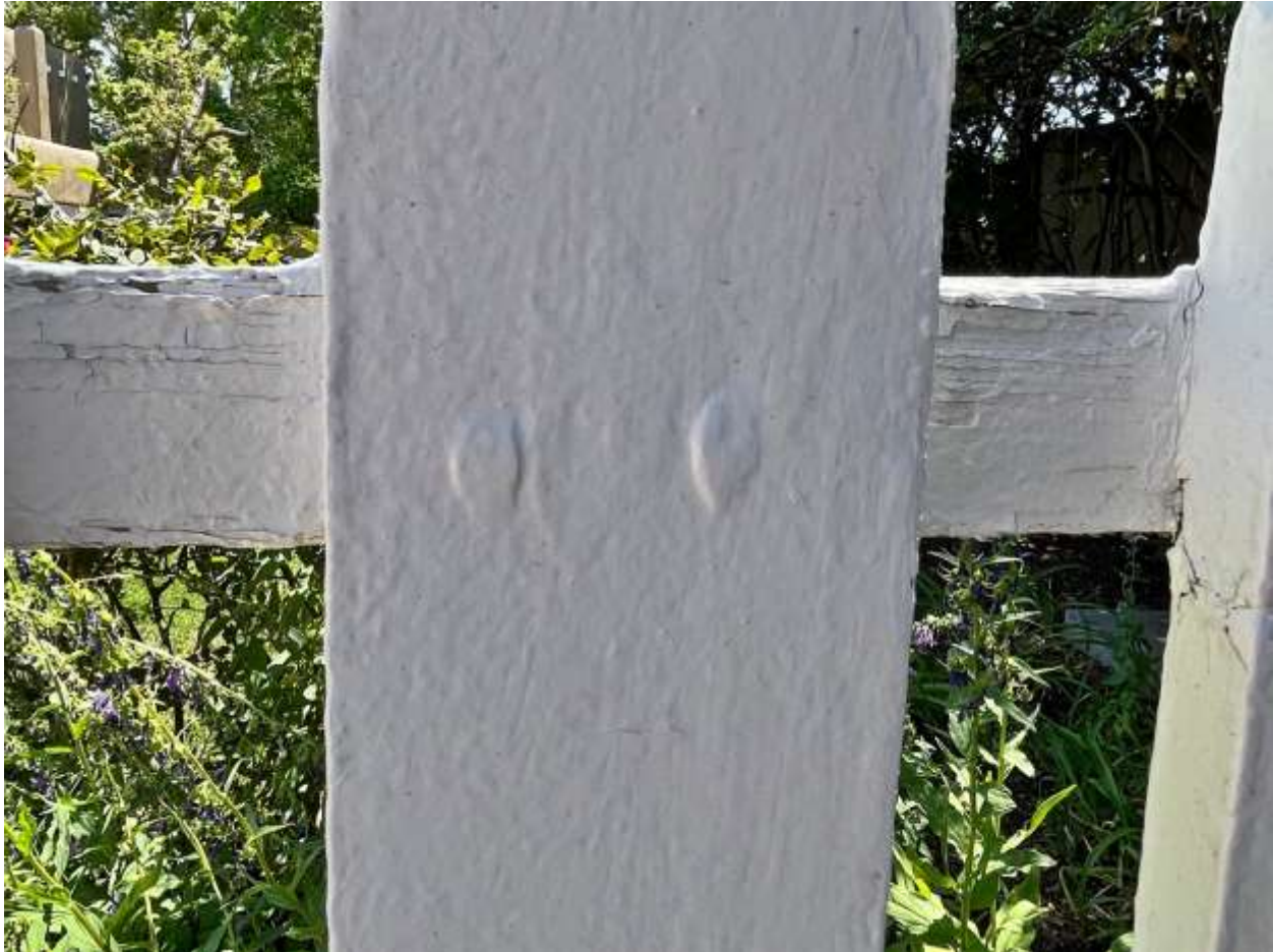
Figure 6: Two-nail pattern on picket. July 25, 2023, John W. Murphey. Note multiple layers of paint on top rail.
