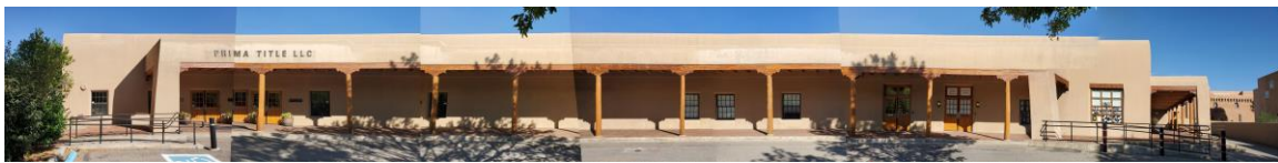
Photo 1: West, front elevation composite shot. Camera facing east. Lorn Tryk: September 3, 2020.
