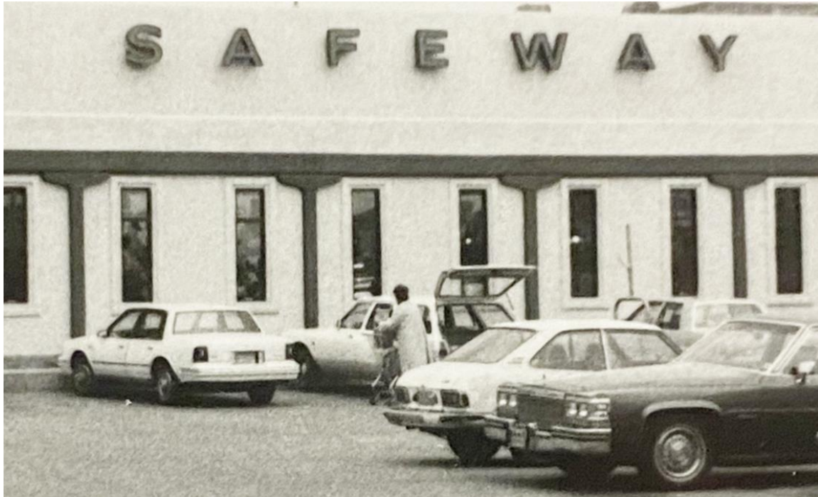
Figure 18: Portion of 1984 photograph of altered Safeway No. 921. Creator: Harry Weiss. Courtesy New Mexico Historic Preservation Division.
