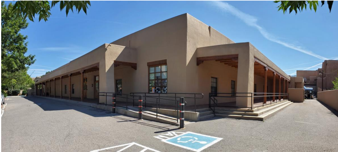
Photo 6: West and south elevations, pantographic shot. Camera facing northeast. Lorn Tryk: September 3, 2020.
