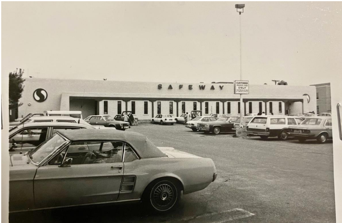
Figure 17: 1984 photograph of altered Safeway No. 921. Creator: Harry Weiss. Courtesy New Mexico Historic Preservation Division.
