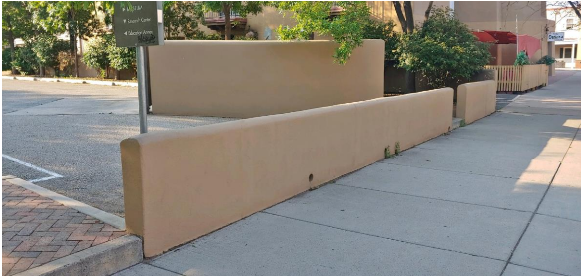
Photo 12: Low walls along Grant Avenue. Camera facing southeast. Robyn Powell: June 13, 2021.
