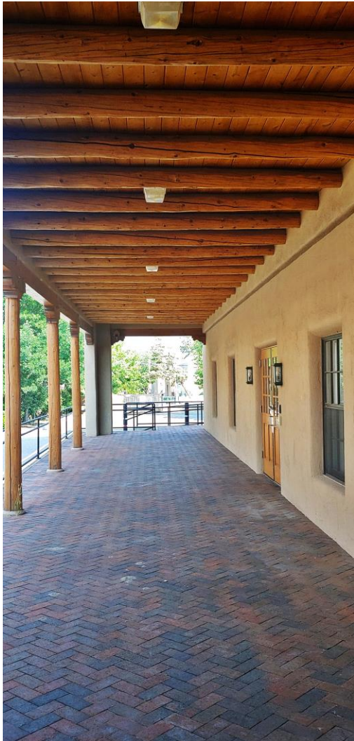
Photo 7: South elevation portal. Camera facing west. Robyn Powell: June 13, 2021.
