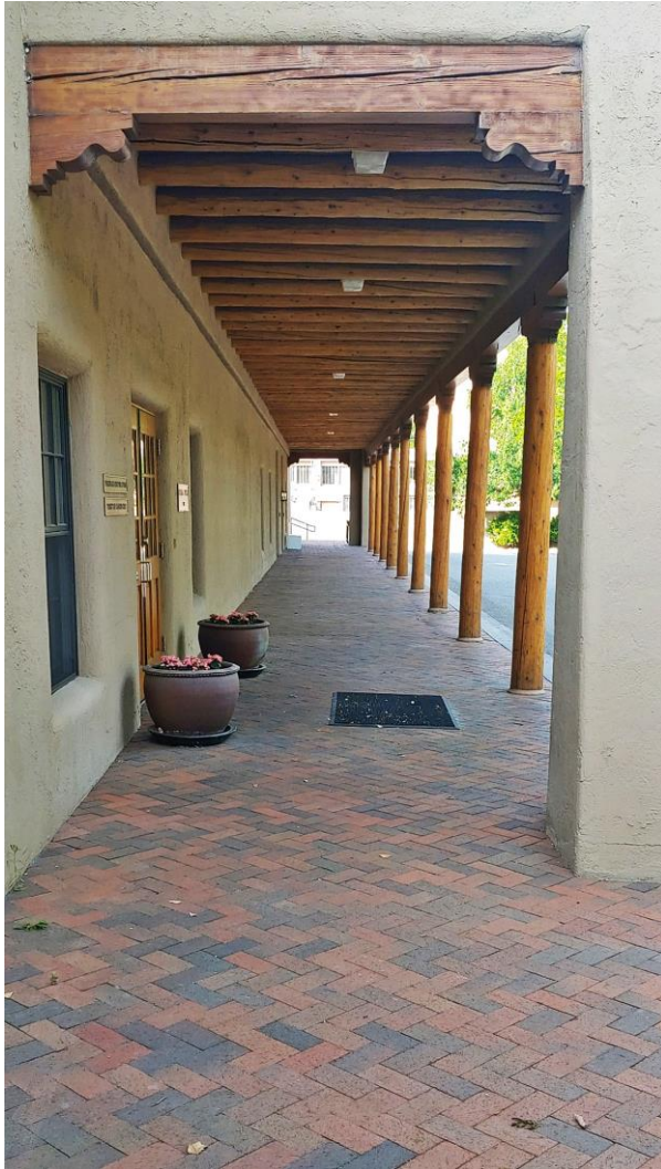
Photo 3: West façade portal. Camera facing south. Robyn Powell: June 13, 2021.
