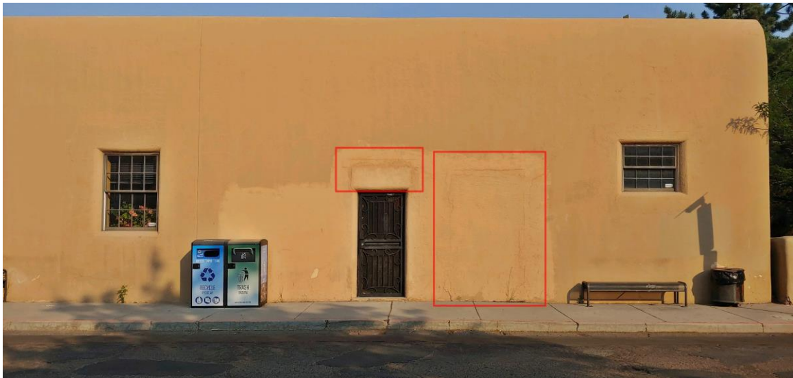
Photo 10: East elevation, north end. Red indicates opening modifications. Camera facing west. Robyn Powell: June 13, 2021.
