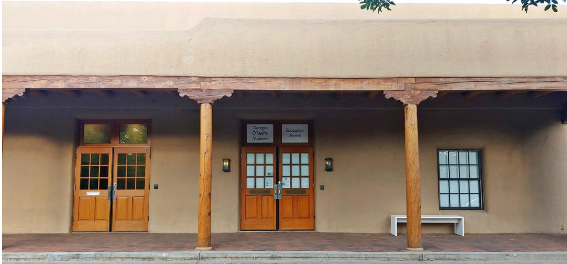
Photo 4: West façade, south end. Camera facing east. Robyn Powell: June 13, 2021.
