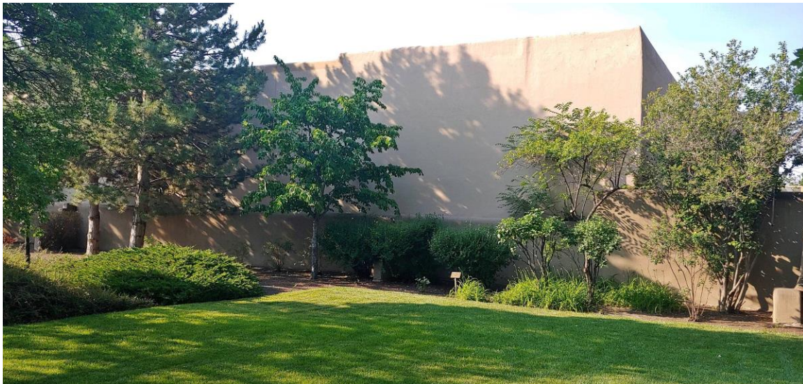
Photo 11: North elevation. Camera facing southwest. Robyn Powell: June 13, 2021.
